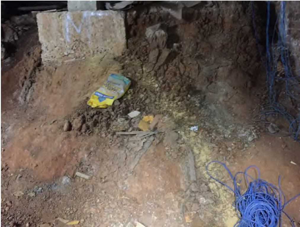
Photo 11: Beneath Block A in Boys High School
