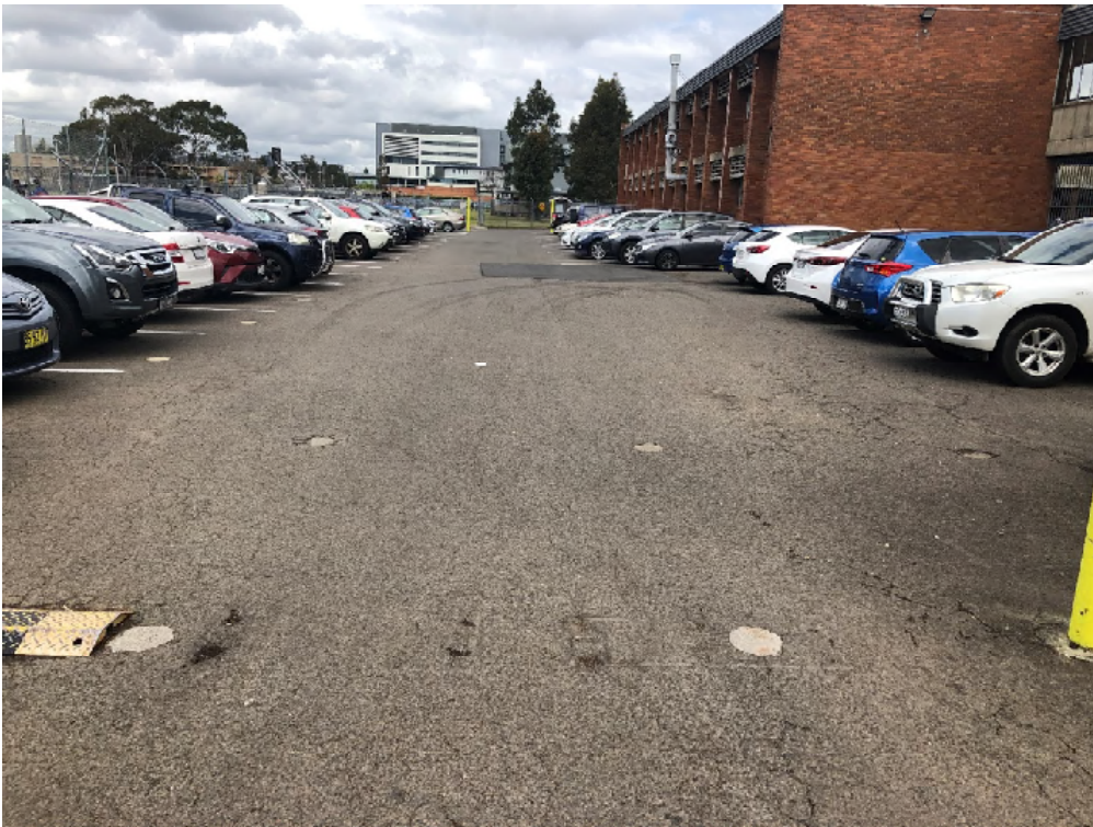
Photo 6. View looking south across Boys High carpark. BH26 is located in foreground.
