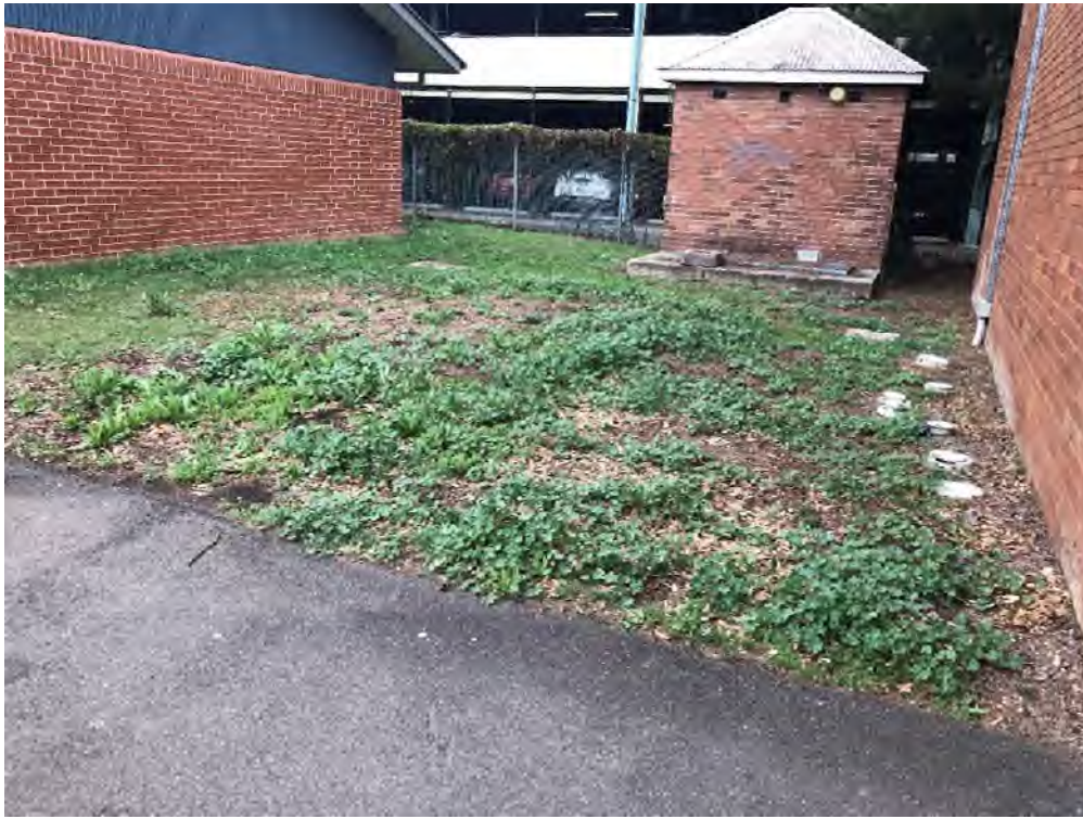
Photo 5. Heritage sewer pumping station located in Girls High on southern boundary
